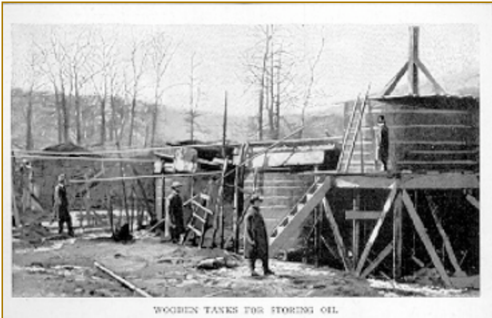
WOODEN TANKS FOR STORING OIL.
